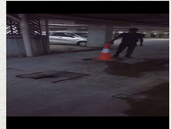
Zinnia Sump pit automation work.
