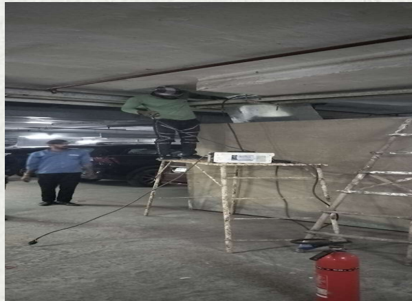
Swimming Pool water supply line from Zinnia Tower
