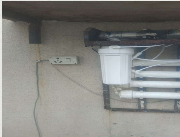
RO system repair work
