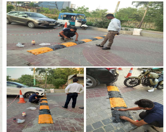
Main Gate Speed Breaker fixing work
